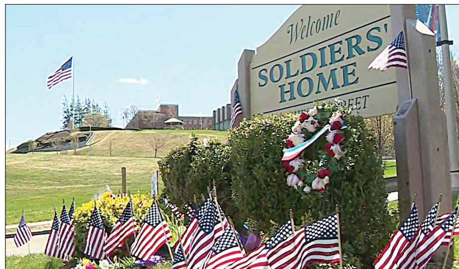
Reconstruction is underway at the Veterans' Home in Holyoke. Federal funding was recently secured for the project. File photo
