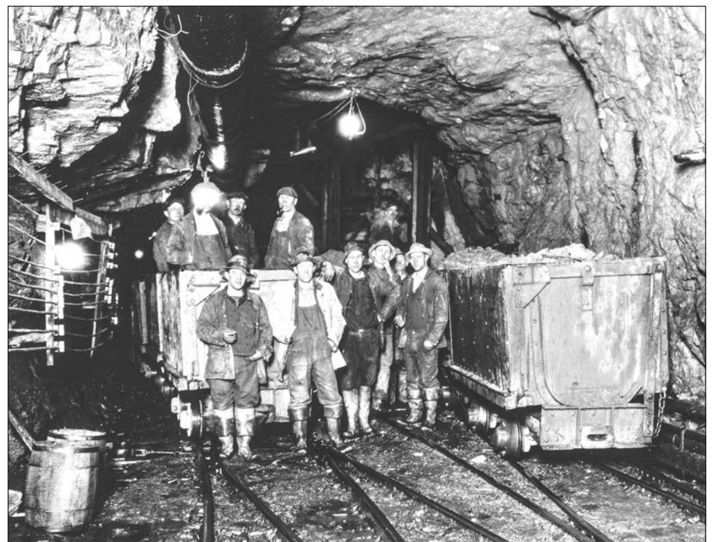
Workers loaded muck cars bottom of shaft #2 depicted during the project showcase the amount of work performed to create the Quabbin Reservoir.
