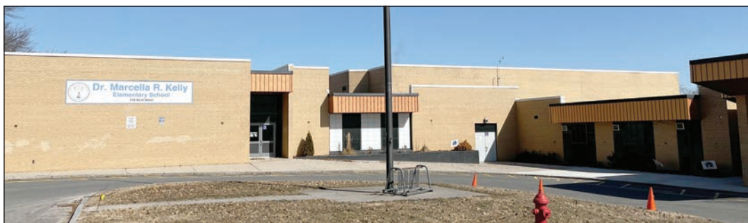
Several school in the city need roof work and the school district is planning to apply to the Massachusetts School Building Authority for assistance.
