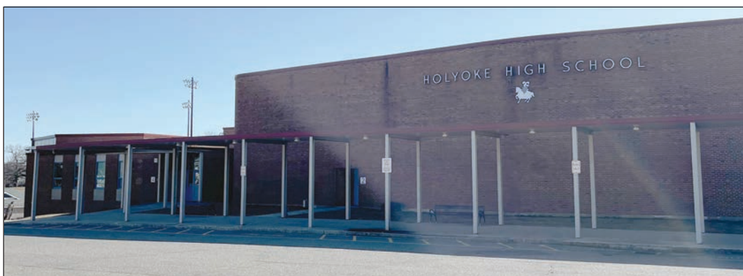
Roof work is needed at Holyoke High School.
