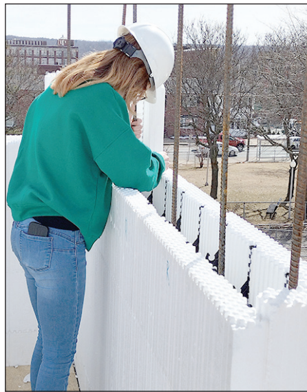
Dean student working with rebar at Chestnut. Submitted photos
